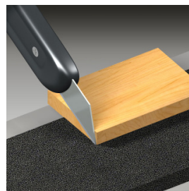
Figure 5: To accommodate setting blocks, notch out tape
