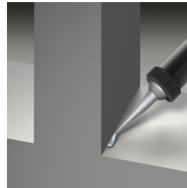
Figure 3: Apply a 10 mm diameter bead of SP525 to bottom corners of the window opening to match joint depth of tape
